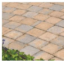
the installation. The Appian® 6"x 6" and 6"x 9" are also available with Natural or Chiseled finishes or a 3" thickness.
