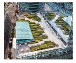
textured Tudor® finish provides slip resistant properties. Safer than gravel ballast, Hanover® pavers make roofs and plazas safe for pedestrians and simplify repairs.
