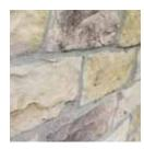
The most common grout technique is a **standard or** raked joint. This is what you typically see with brickwork, for example. The grout is evenly applied around the edge of each stone or brick. When finished,
